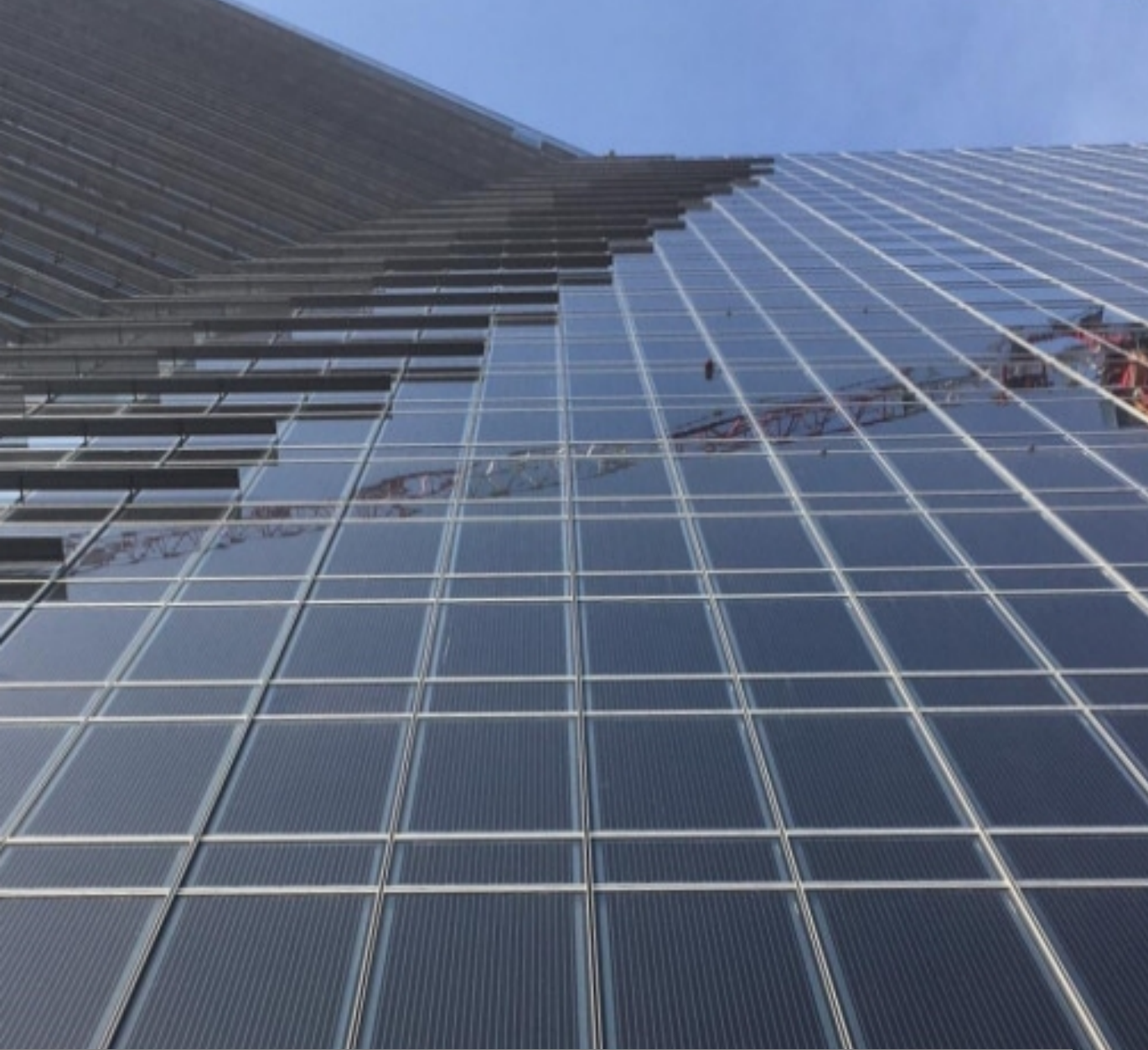
Mono-Crystalline Silicon Technology in Spandrel area Gioia 22 Tower, Porta Nuova , Milan - Italy
