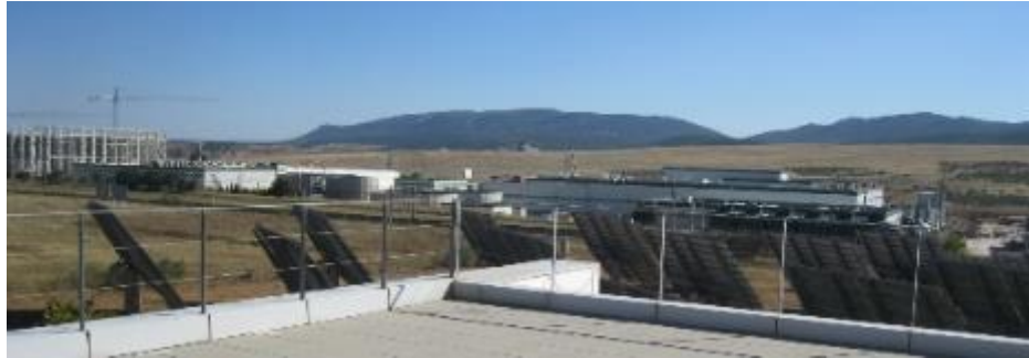
Figure 2.7: ISFOC rooftop balustrade
