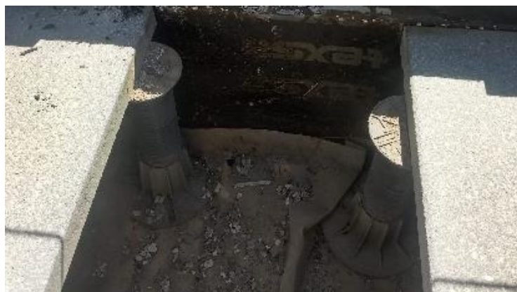
Figure 2.11: Detail of the supporting elements (plots)
