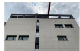
picture house A, north-east facade
