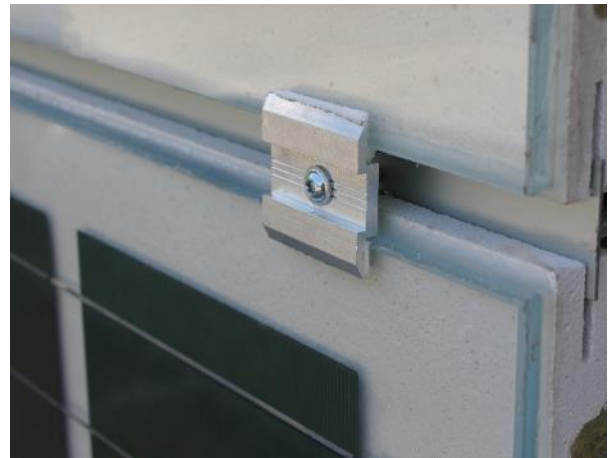
Figure 5.19: Demo-site 4, Middle safety clamp
