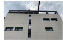
picture house A, north-east facade
