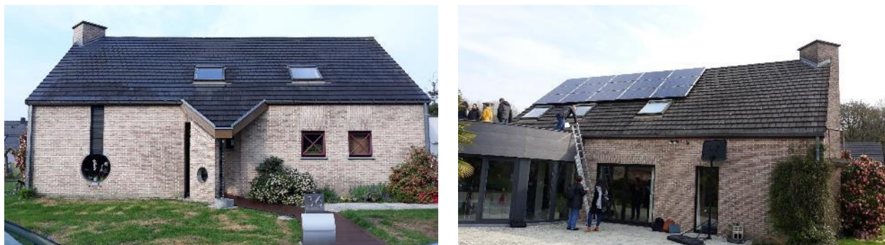
Figure 4.7: Demo-site 3 building, east and west side
