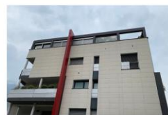
picture house A, south-west facade
