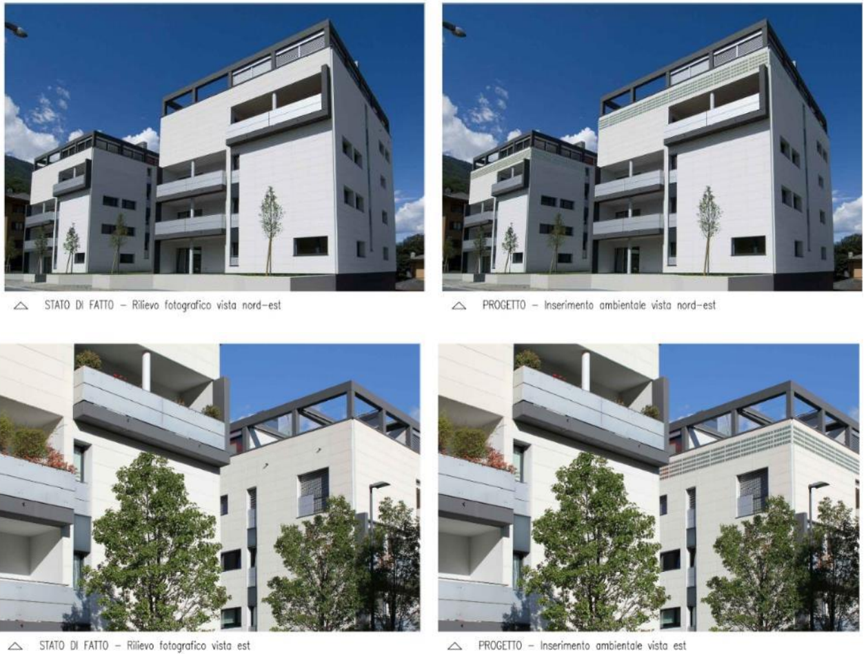
Figure 5.11: Demo-site 4, 3D design of demo-site building design with and without ePIZ BIPV modules
