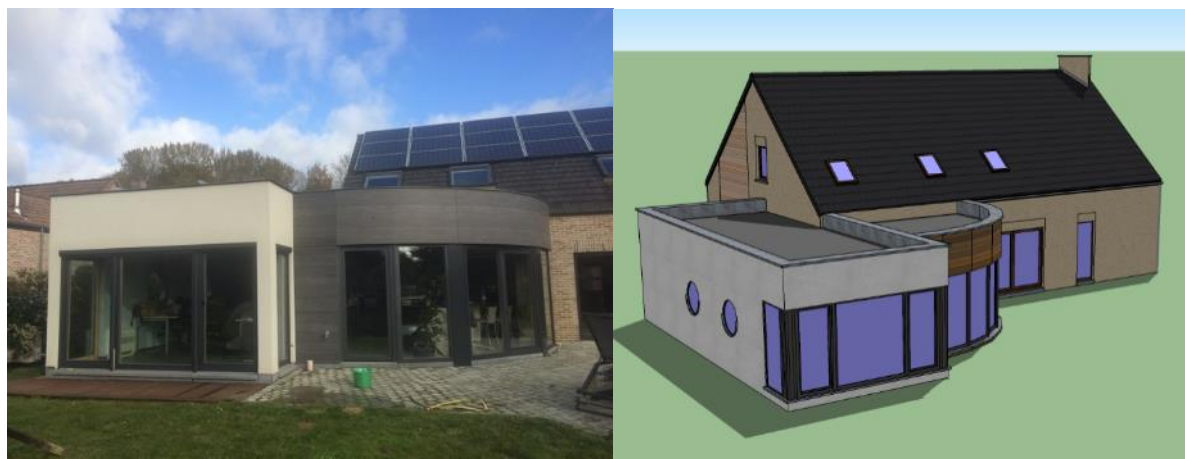
Figure 4.3: Picture of the office next to the house (left) and top view of the whole building (right)
