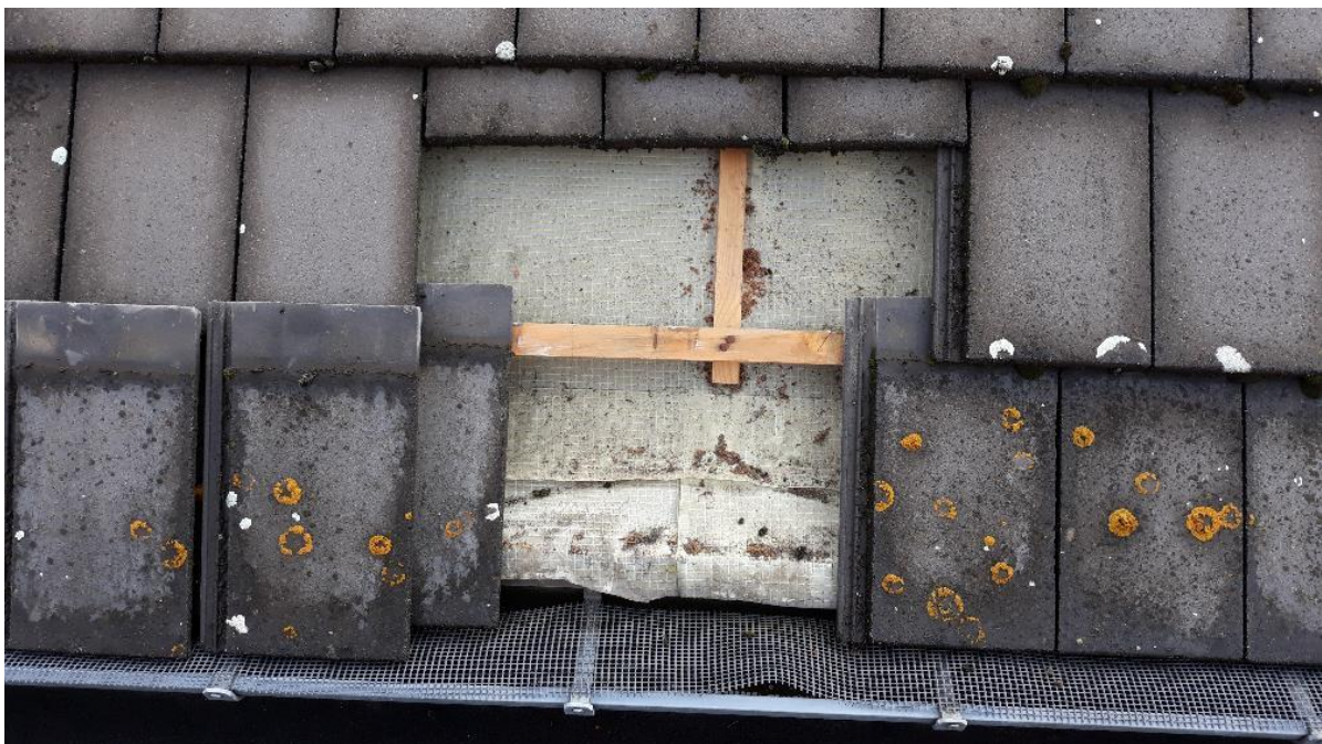
Figure 4.24: Existing roof structure of Demo-site 3
