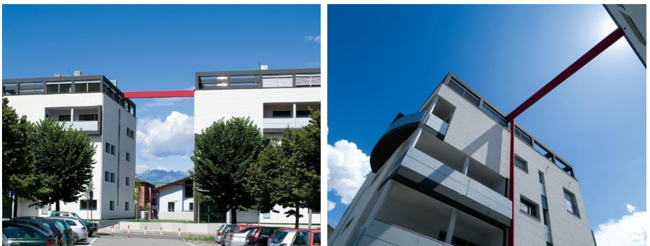
Figure 5.2: Demo-site 4, Images of the building
