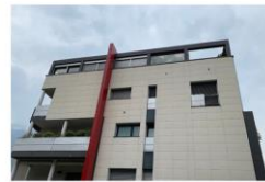
picture house A, south-west facade
