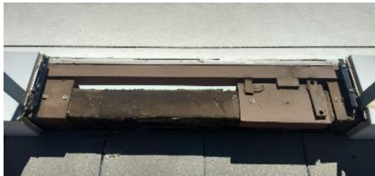
Figure 2.9: Attachment of the balustrade to ISFOC building
