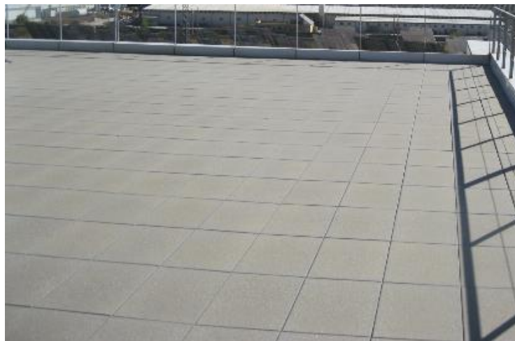
Figure 2.10: ISFOC walkable floor, concrete tiles
