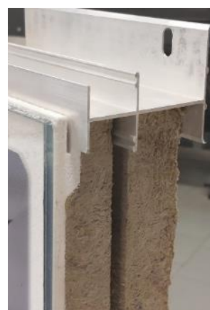
Figure 5.17: Demo-site 4, Aluminum H-profile placed inside the upper horizontal grooves
