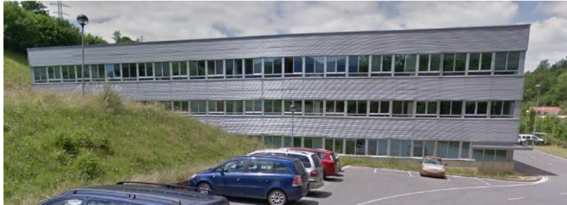
Figure 3.3: East façade of MASS building
