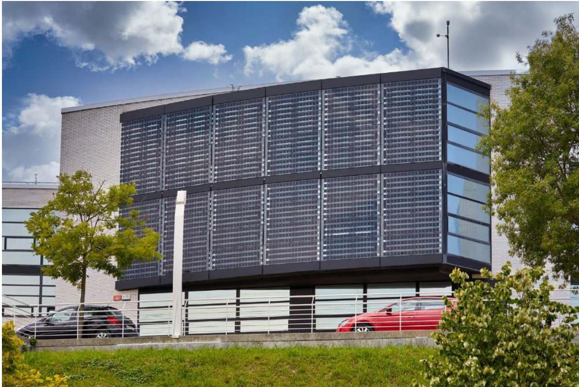
Credits: TECNALIA, PVsites project
