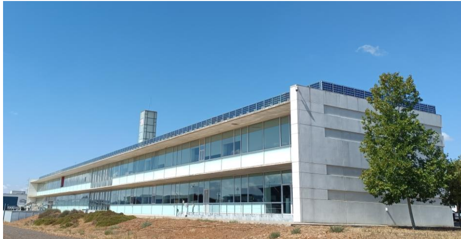
Figure 2.1. Demonstration site 1 – BIPV balustrade. South and east facades view from the ground level
