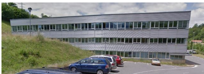
Figure 2.13 East façade of MASS building
