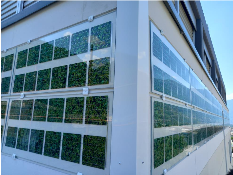
Figure 2.31: Corner view of multifunctional BIPV cladding system
