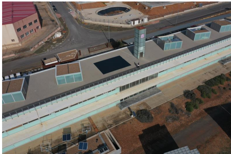
Figure 2.10. General view of ISFOC's rooftop, walkable floor location
