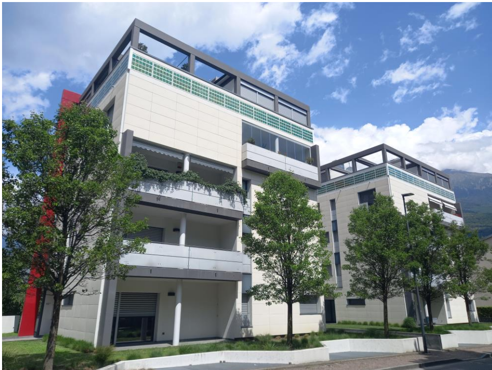
Figure 2.32: Demonstration site 4, South-East view
