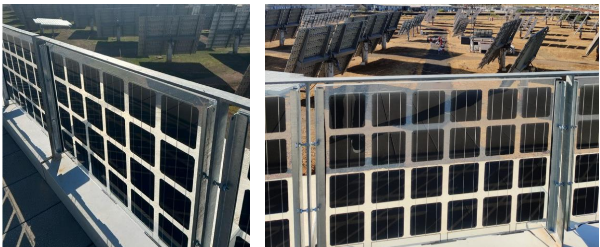
Figure 2.5. Detail of the BIPV modules installed in the balustrade
