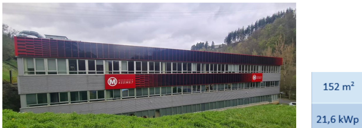
Figure 2.22 Final Demo2 Façade
