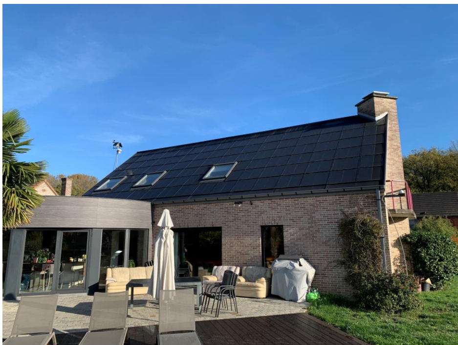
Figure 2.24: Demonstration site 3, West view
