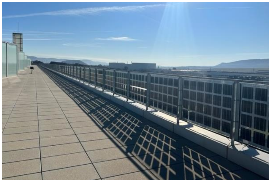
Figure 2.2. South balustrade view from the rooftop
