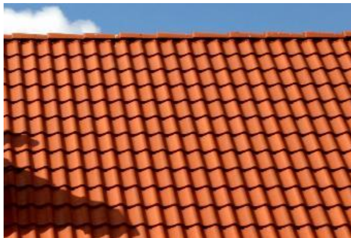
Roof with ceramic tiles
