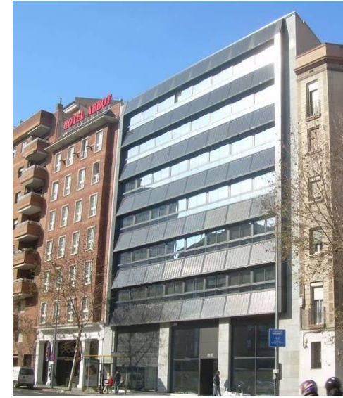
COMSA INDUSTRIAL, BCN. 22 kWp (2014)
