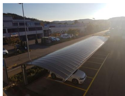
Figure 14 Carport, Flisom, roof, CH
