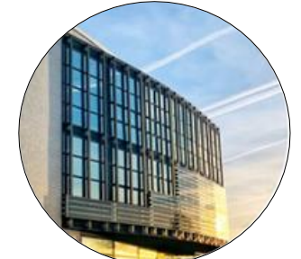
Enhanced, cost effective BIPV roof and facades systems for CIGS on metal and c-Si glass-glass
