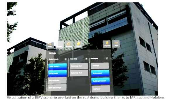
Visualization of a BIPV scenario overlaid on the real demo building thanks to MR app and HoloLens
